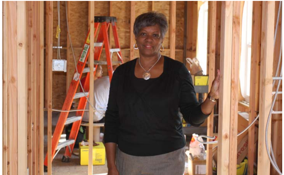
Clara Perkins, director of the S.A.Y. Yes! after-school program, stands in the doorway of her new office in the facility under construction.
